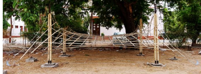
Figure 5. Doubly curved shell with square grid
