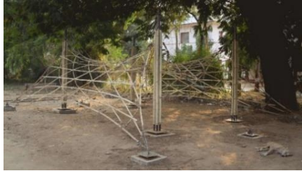
Figure 4. Doubly curved shell with diagonal grid
