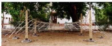
Figure 2. Doubly-curved Shell with square grid
